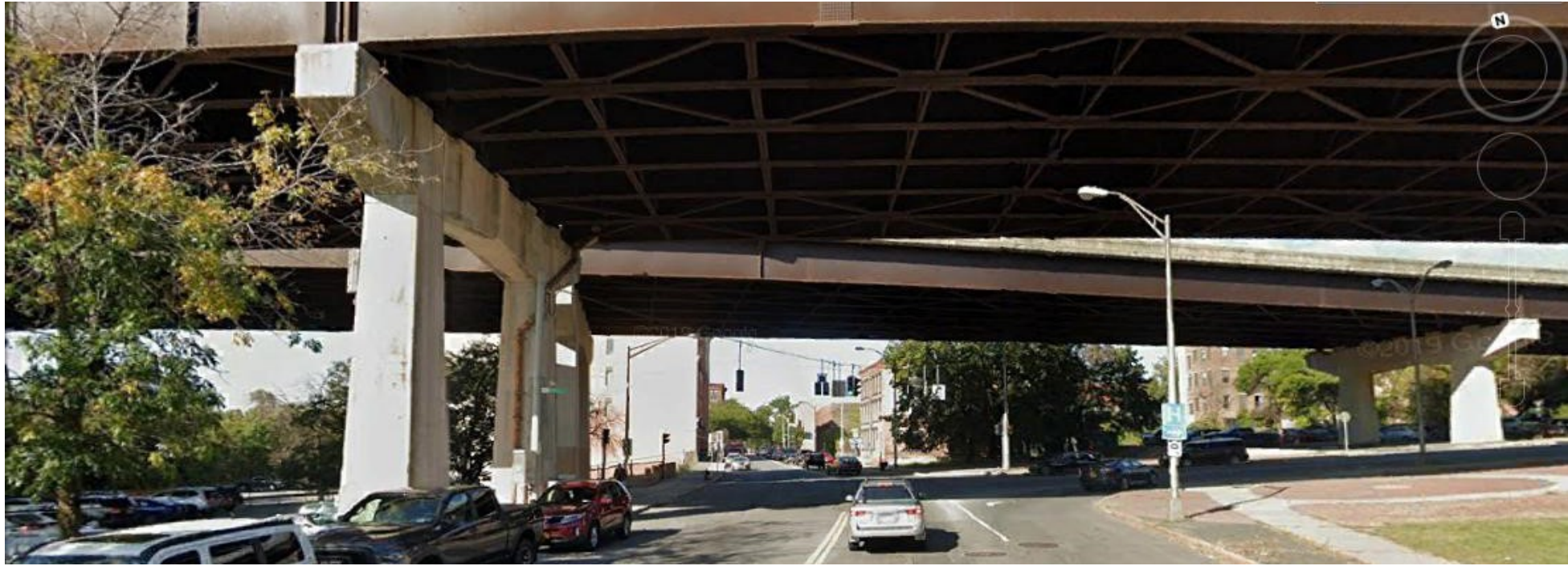
VIEW NORTH UP RIVER STREET TOWARD TROY'S MOST DISTRESSED NEIGHBORHOODS.
