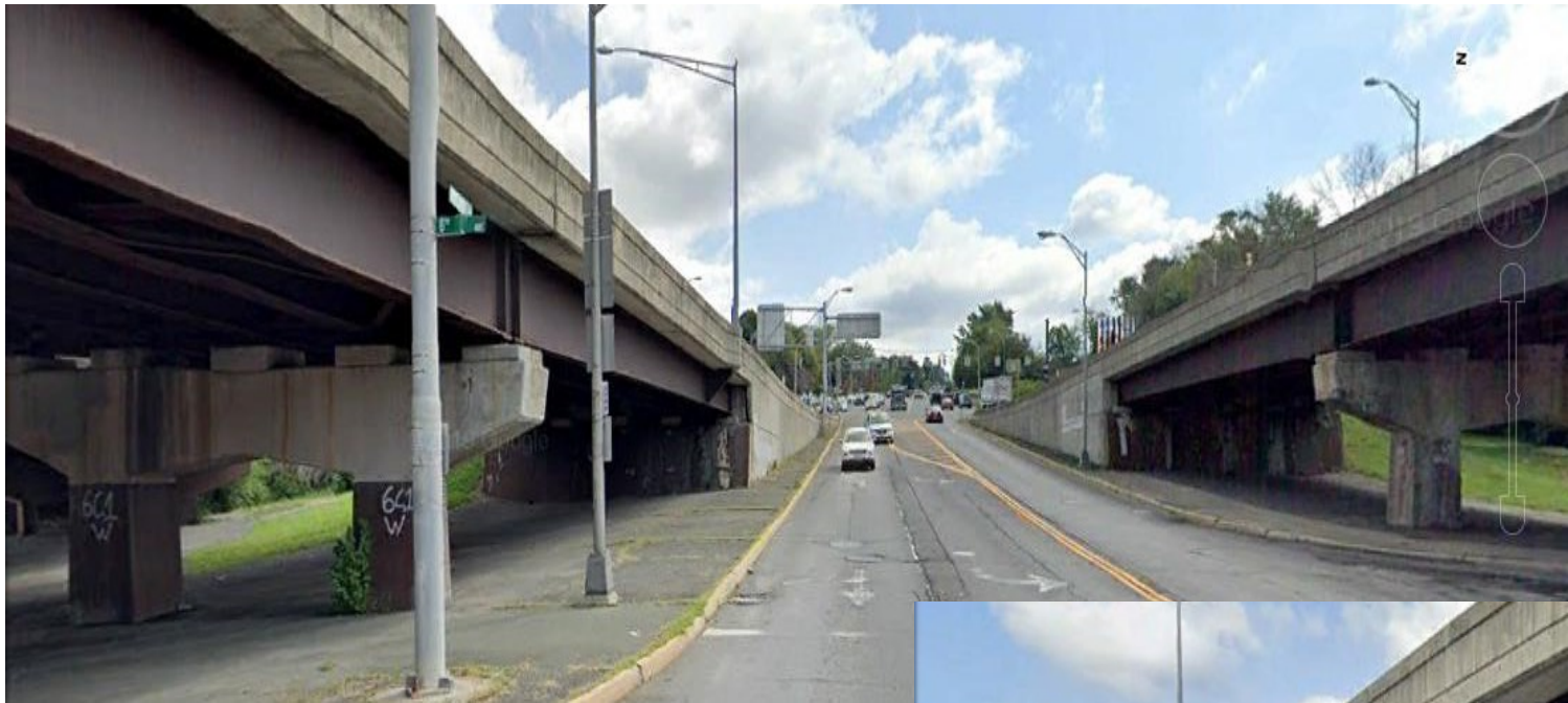
VIEW EAST UP HOOSICK STREET AT 6TH AVENUE
