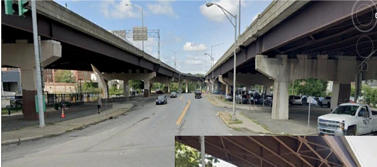
VIEW WEST DOWN HOOSICK STREET AT 6TH AVENUE
